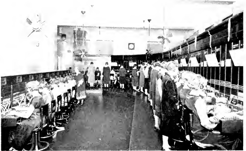
INSTRUCTING STUDENT CENTRAL OFFICE OPERATORS AT PRACTICE SWITCHBOARDS
